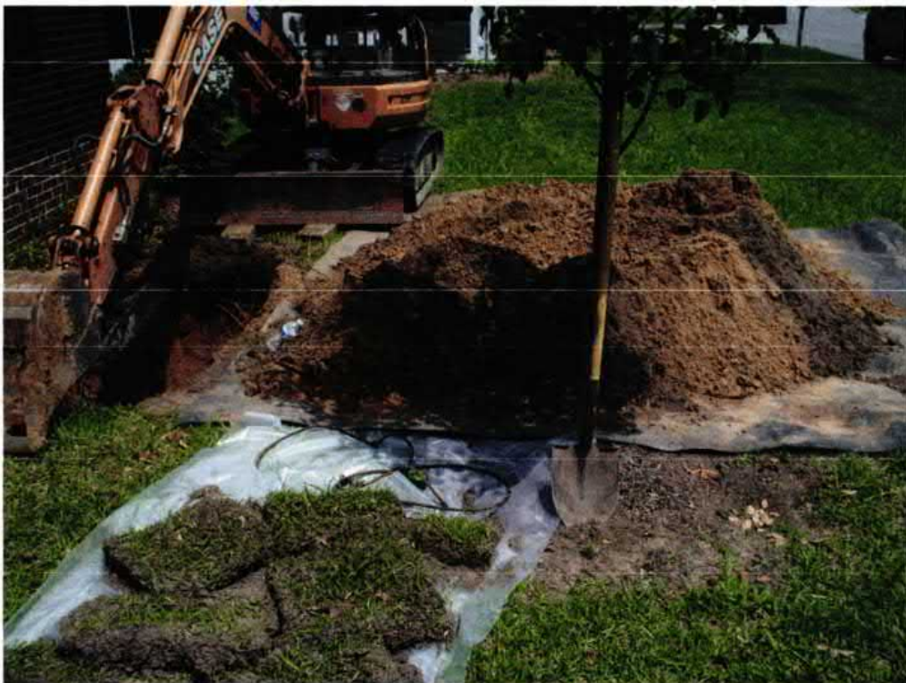
Picture 2: UST 854Dolphin excavation in progress.
